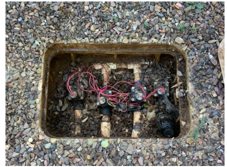
Irrigation valves - Rear
