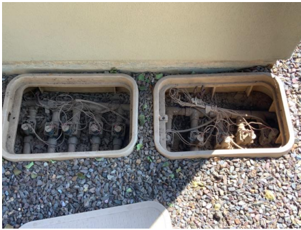
Irrigation valves - Front
