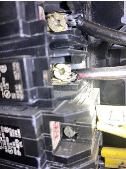
Damaged connections sub D
